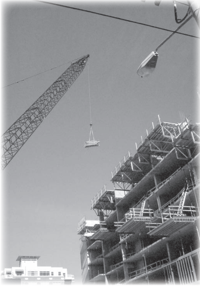
Construction scenes remain common across the region.
